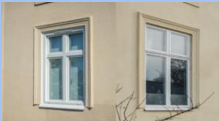
Before and after a window replacement - t.r. a new aluminium window t.l. the old wood window. Photo of a building in Nyköping, taken by David Hansson, Sörmlands museum.
