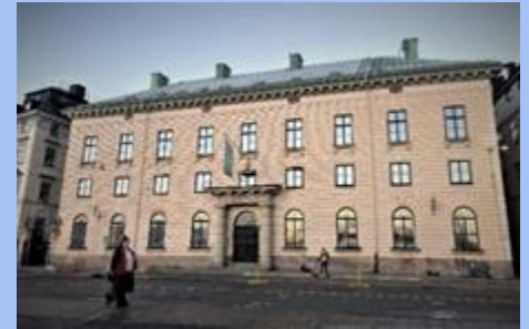
Above Generalltullstyrelsens the Old Town of Stockholm , picture taken 1930-1940 by Lennart af Petersens, Stockholmskällan. Below the same building an early november morning in 2020. The building has undergone became 20 % more energy efficient since the property owner added 1000 extra insulating glass. See Goda exempel, Spara och bevara.
